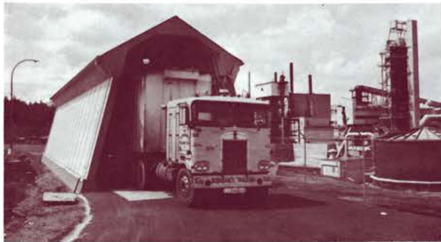
The new weighing station for trucks hauling chips to Harmac. The up-to-the-minute weigh-scale automatically produces weigh-tickets with the name of the supplier, the truck and load number and the chip species, as well as the weight of the load. [The driver of the truck in the picture doesn't show up too well, but it's Grant McAlpine, of Dorman's.]
