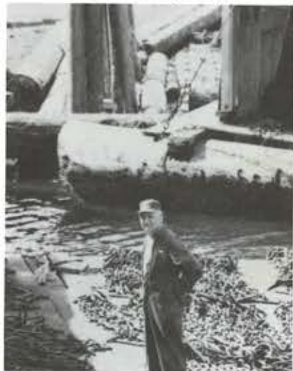
Chainman George Copley surrounded by some of those large chains that hold the booms together. The chains weigh anywhere from 30-85 lbs. apiece.
